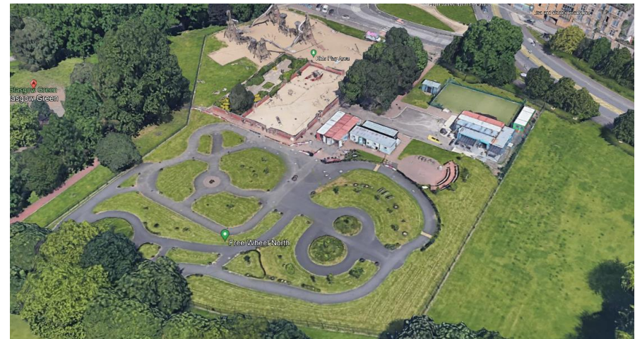
Cycling Track and Associated Buildings on Glasgow Green
